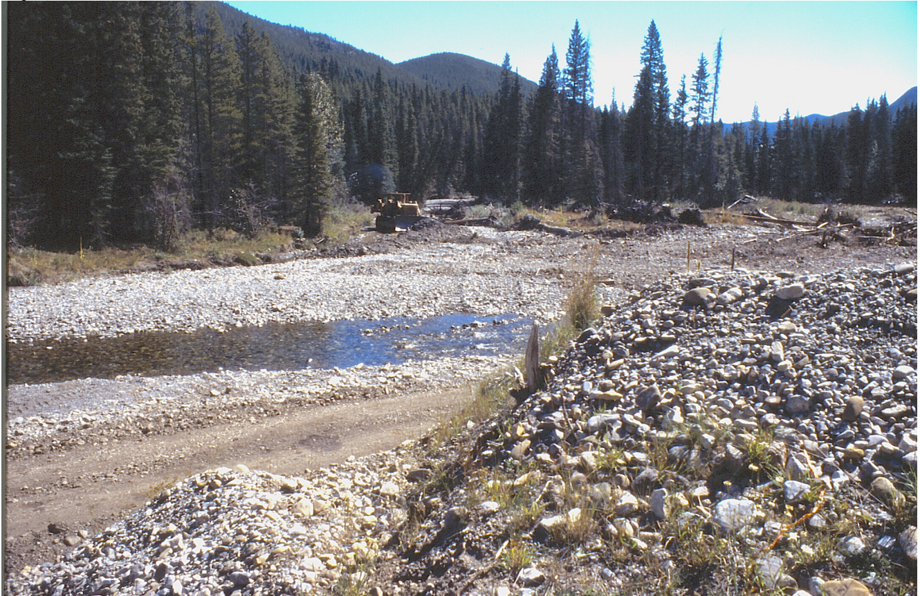
Figure 2. New, shorter channel (background) being constructed for Lynx Creek, now in a reach that is critical habitat for westslope cutthroat trout, to accommodate the Sartoris Road (foreground) in the natural channel. September 1998.
